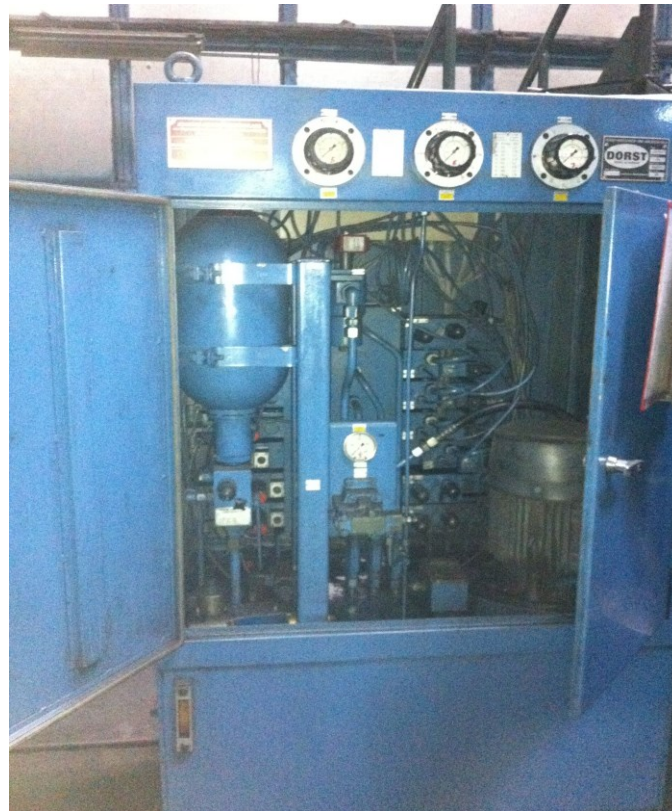
Hydraulic aggregate of TPA 50 to (for hydraulic study)
